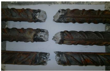
Failures of G2 25mm bars
