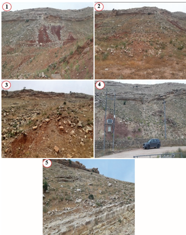
Fig. 6. Right bank station Nos. 1, 2, 3, 4, and 5. Nos. 1 and 4: Active erosion areas indicating unstable slopes. No. 2: Bulged mass in the middle of the slope indicating an unstable slope. No. 3: Recent slid blocks as indicated from the fresh color of the blocks; indicating unstable slope. No. 5: The slope below the cliff is gentler as compared to the other stations; therefore, the amount of slid blocks is smaller and lesser. The reddish brown clastics of the Gercus Formation are overlain by the carbonates of the Pila Spi formation
