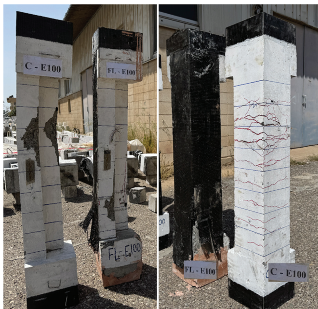
Fig. 8. Mode of failure and crack pattern of column specimens ( e_x = e_y = 100 mm).
