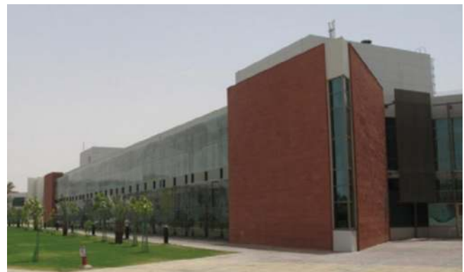
Fig. 15. Arch. Engineering Department in UAE University, Al-Ain City (Radhi, Sharples and Fikiry, 2013).
