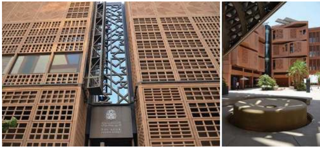
Fig. 20. Modern interpretations of the Islamic Mashrabiya. Left, The Souk and right, Masdar City, located in Abu Dhabi, UAE. By Foster + Partners. (Boake, et al., 2014).
