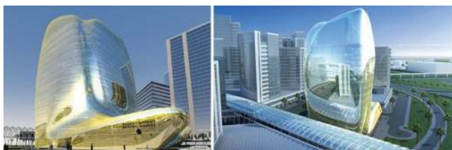
Fig. 8. External views of National Holding's building (right: Yagoub, Appleton and Stevens, 2010) (left: Wallner and Pottman, 2011).
